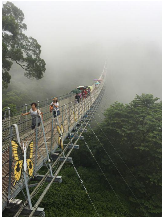
Salon HM - Potse Chen, Taiwan, Bridge View
